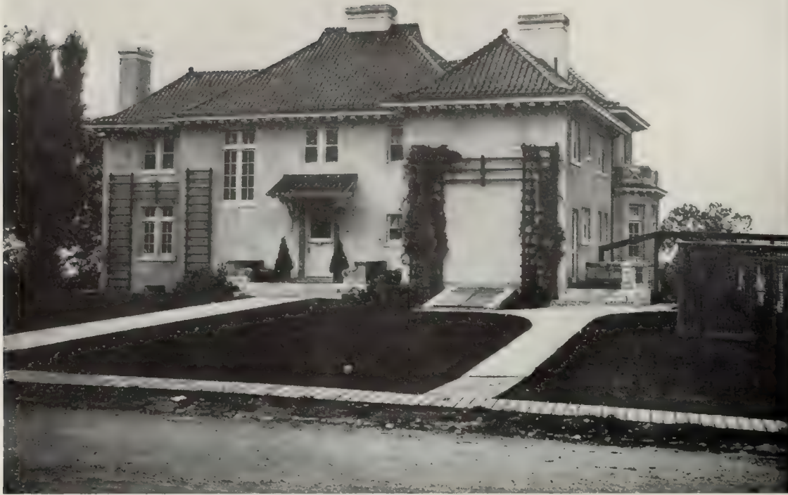
WESSON HOUSE FROM STREET
